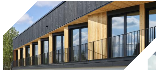
Modular and circular construction, Nei Schmelz, Dudelange
