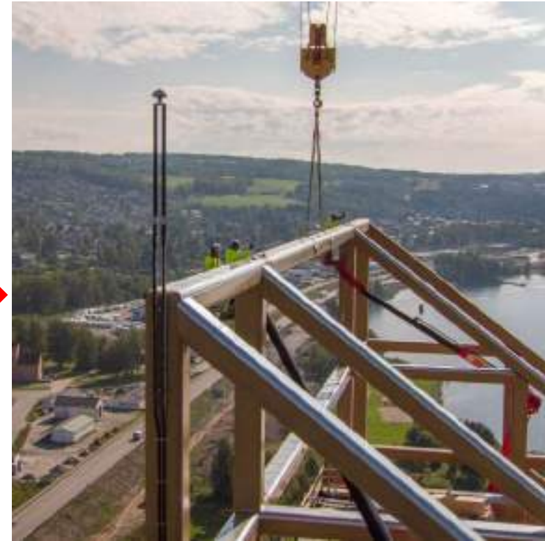
4th September 2018 Last beam
