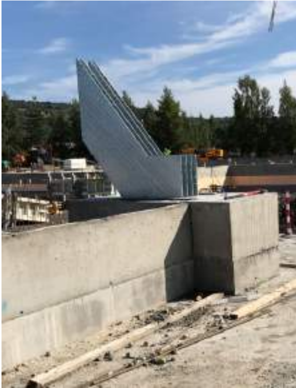
July 2017 Positioning anchor plates
